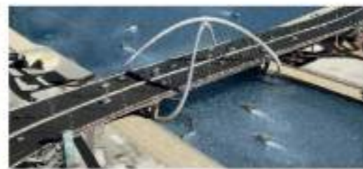
Shindagha Bridge – Dubai
